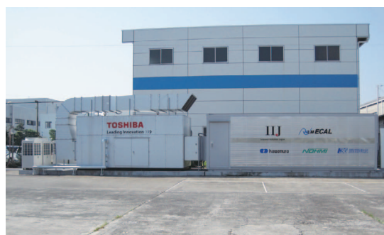
Figure 9: From Left - Outdoor Compressor Units, Cooling Module, and IT Module
