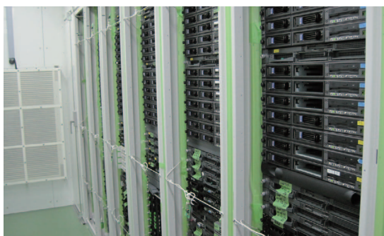
Figure 10: Masking Tape Applied Between Racks to Raise Cooling Efficiency
