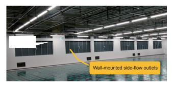
Figure 11: Side-flow Air Conditioner Outlets
