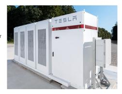
High-capacity lithium-ion batteries installed at the Shiroi DCC
