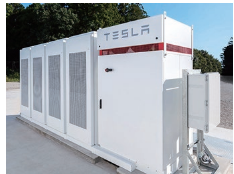
High-capacity lithium-ion batteries installed at the Shiroy DCC
